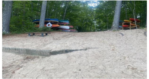
Steep grade leading from parking area directly to pond, showing overtopped, wooden retaining wall.
