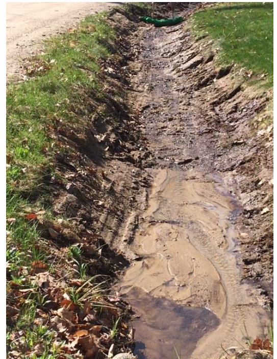
Road ditch maintenance causing erosion on Avon Shores Rd, May 2022. Photo credit: Kevin Kelly.
