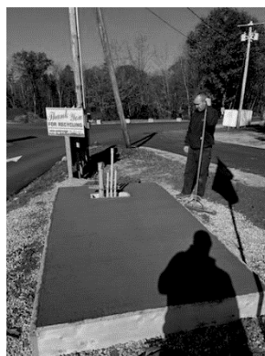
Installation of the new Transfer Station generator pad;
