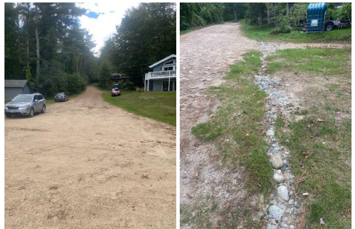
(Left) Steep grade leading directly to beach area/lake, (Right) eroded left side of road running off into gully.
