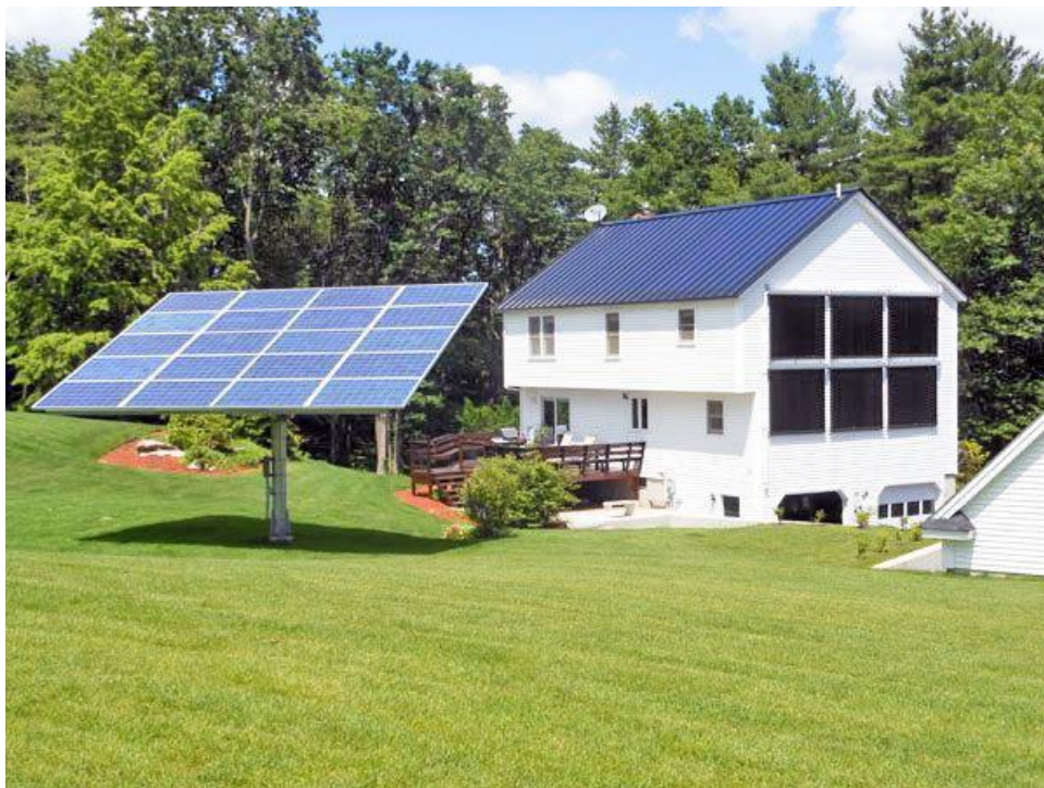
Tracker Mounted Residential System: Courtesy Revision Energy
