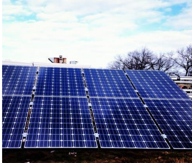
Completed installation showing gaps between panels
