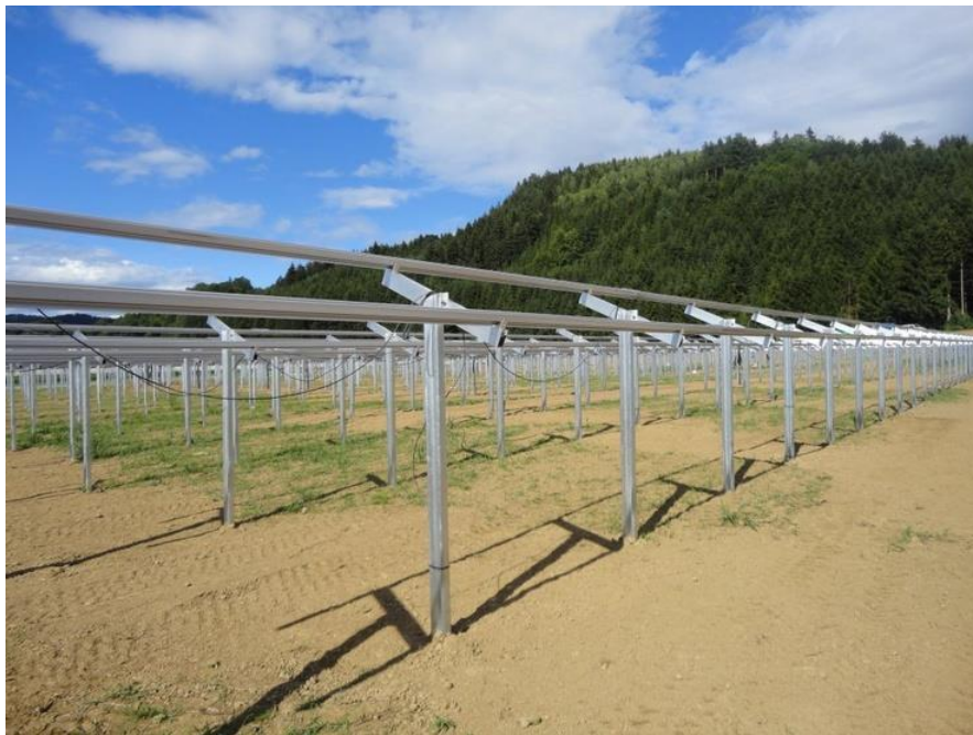
Racking equipment – prior to panel installation.
