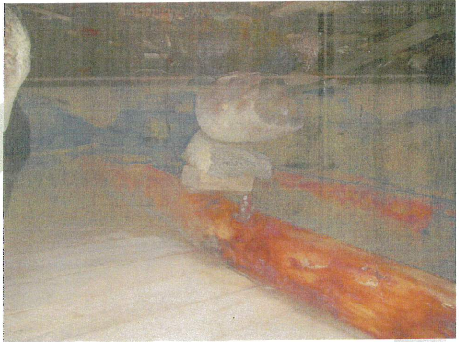
Photo: 32 Location: Taylor-French House 970 Whittier HW Moultonborough, NH Date: August 3, 2017 Description: Falling Stacked Rock Post at Barn
