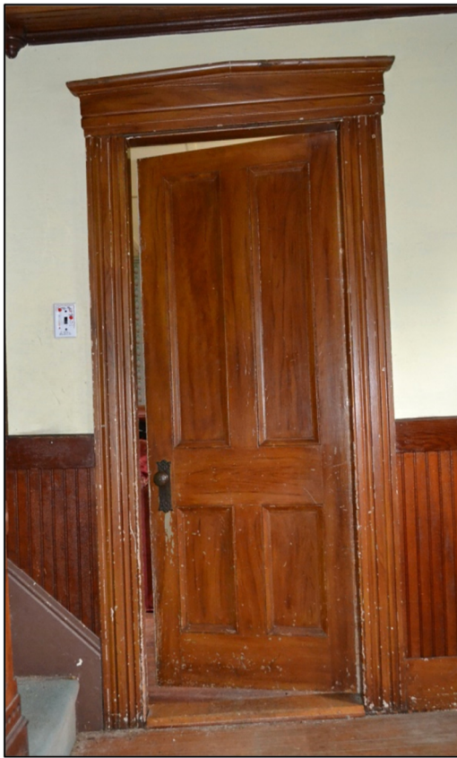
Left: Original door with graining, hardware and adjacent wainscoting added circa 1900. Right: Detail of original door casing and entablature.
