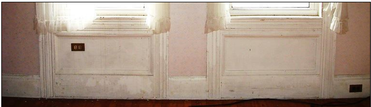
Above: Plaster panels with wooden trim below first-story windows. Photo by Cristina M. Ashjian.
