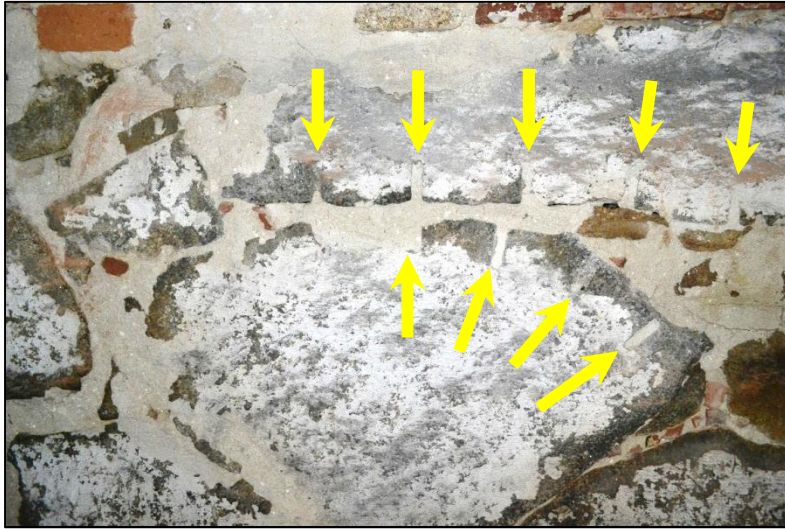
Above: Basement wall, showing the marks of plug drills.
