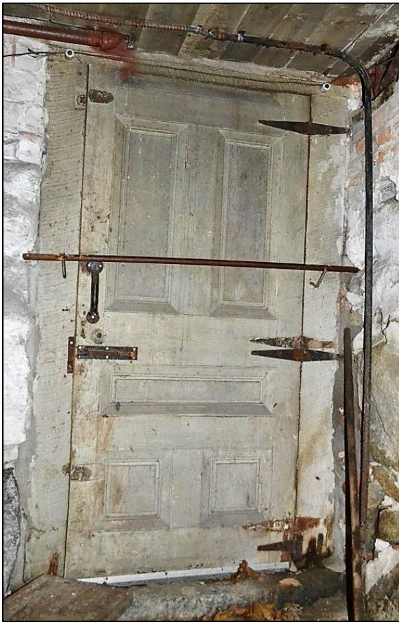
Left: Exterior door re-used in cellar. Note that the upper panel has been cut off.
