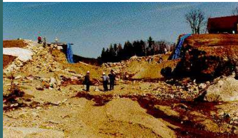
Alton dam breach, 1996
